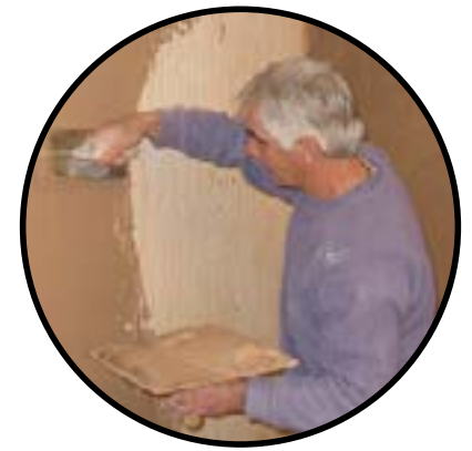
Picture shows a plasterer covering a wall, using a traditional plasterer's hawk (in his left hand) and applying the plaster off the hawk onto the wall with the trowel.
